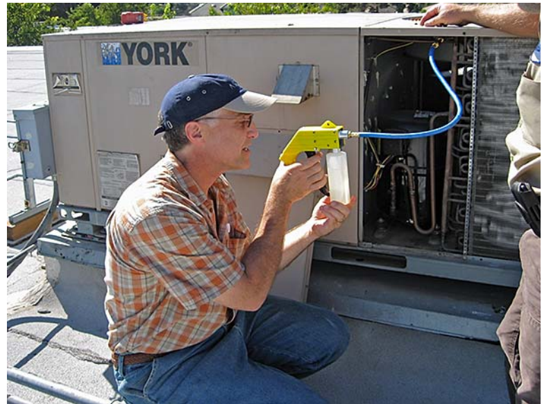
Figure 4. Installing the Synthetic Refrigerant Catalyst
